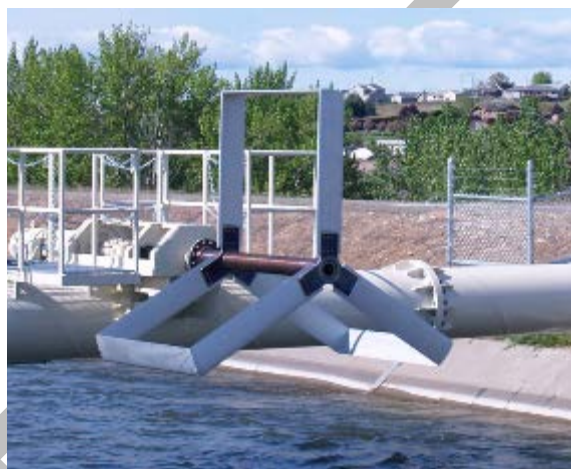
Figure 51. Energy, Roza Canal, Oregon. Source: Instream Energy https://www.instreamenergy.com/yakima-washington
