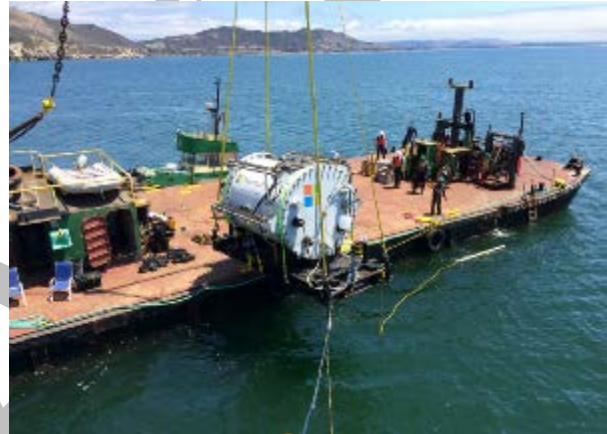
Figure 47. Microsoft Project Natick – modular submersed server with ocean cooling, San Luis Obispo, California. Source: Microsoft
