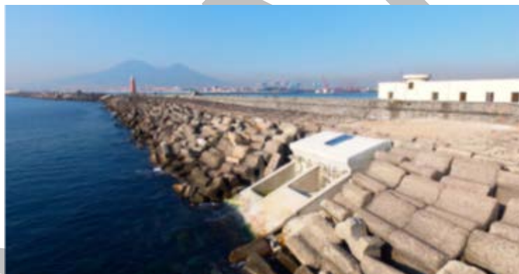
Figure 56. Overtopping breakwater for energy conversion prototype in Naples, Italy. Photo from Contestabile et al. (2017)
