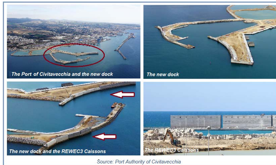
Figure 55. The Resonant Wave Energy Converter 3 Device in Civitavecchia Port, Italy. Photos from Maestrale
