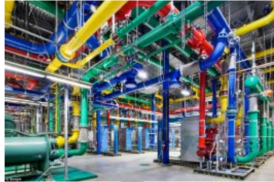
Figure 46. Google data center with closed-loop water cooling in Hamina, Finland. Source: Google
