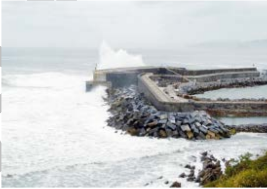
Figure 54. Mutriku, Spain, breakwater-OWC integration. Photo from TidalEnergy Today
