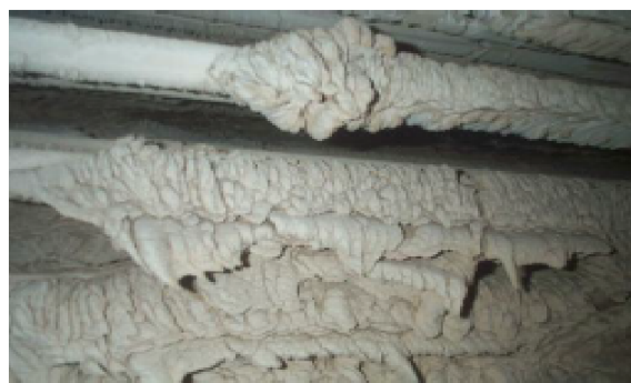
Figure 4–5 Secondary super heater fouling: potassium sulfate (left); potassium chloride (right).
