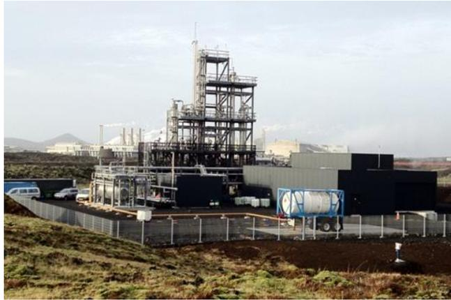
*Figure D7: George Olah geothermal-to-methanol plant utilizing hydrogen from water electrolysis<sup>104</sup>*
