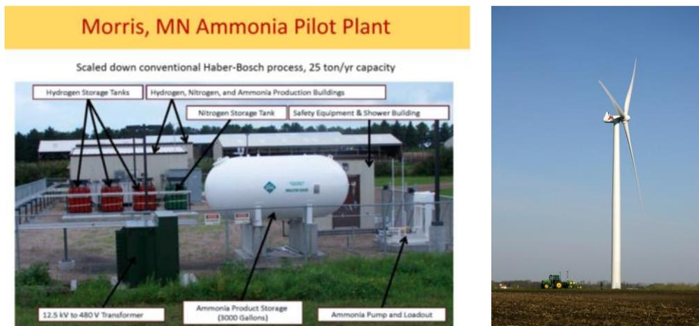
Figure D6: Wind-to-Ammonia project showing  $\text{NH}_3$  production facility and wind turbine<sup>102</sup>
